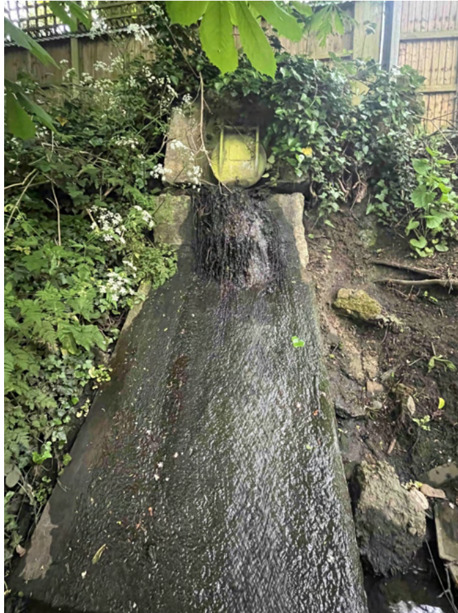
Figure 3b. Example of a utilities polluting outfall. Lennox Estate BEVB0025 (score = 4).
