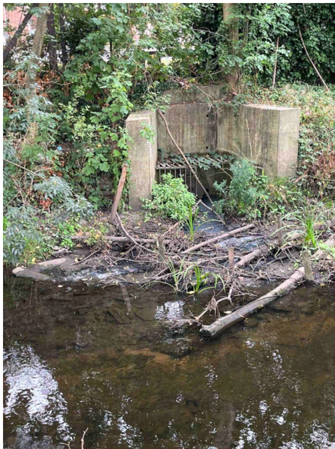
Figure 3b. Example of a utilities polluting outfall. Lennox Estate BEVB0025 (score = 4).
