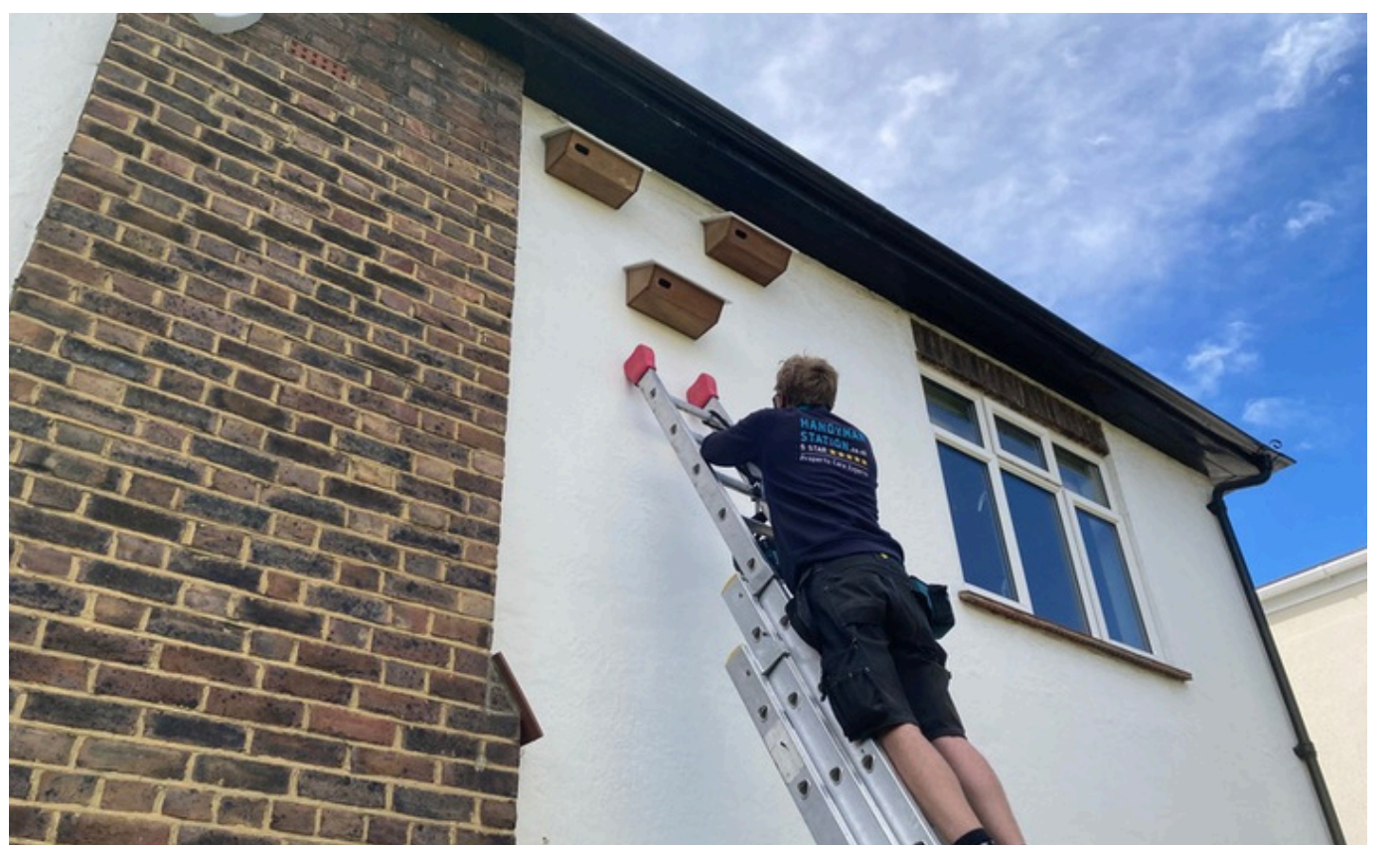
Jeremy from Handyman Station installing 3 swift boxes
